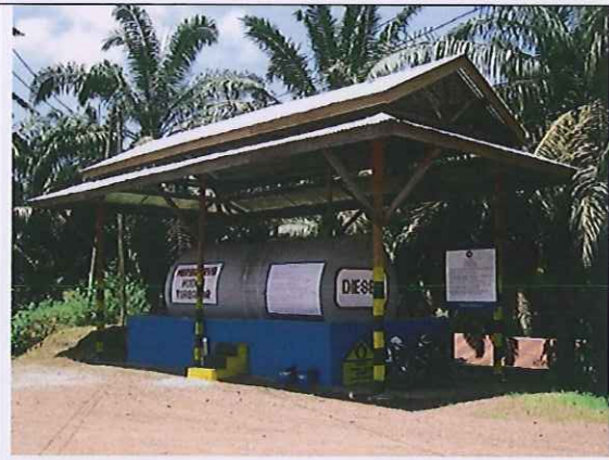
Bunding provided for the diesel tank.
