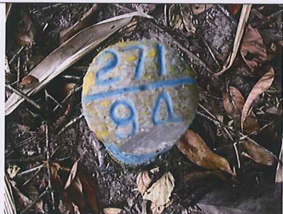
Verification of boundary stone markings
