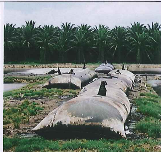
Hydro K tubes used at the effluent ponds at POM.
